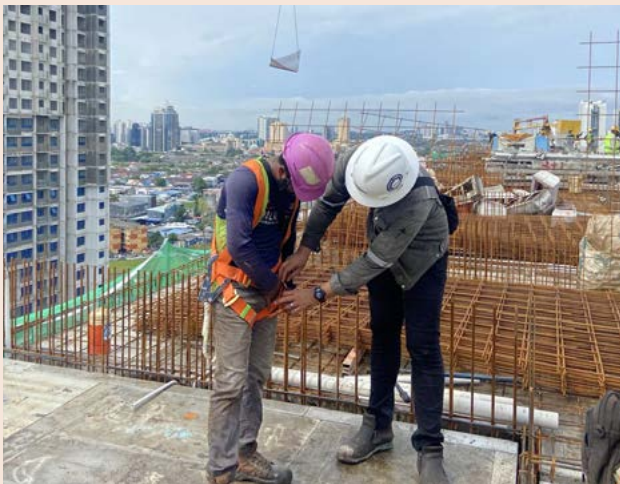
Worker training on the use of safety harness for working at height
