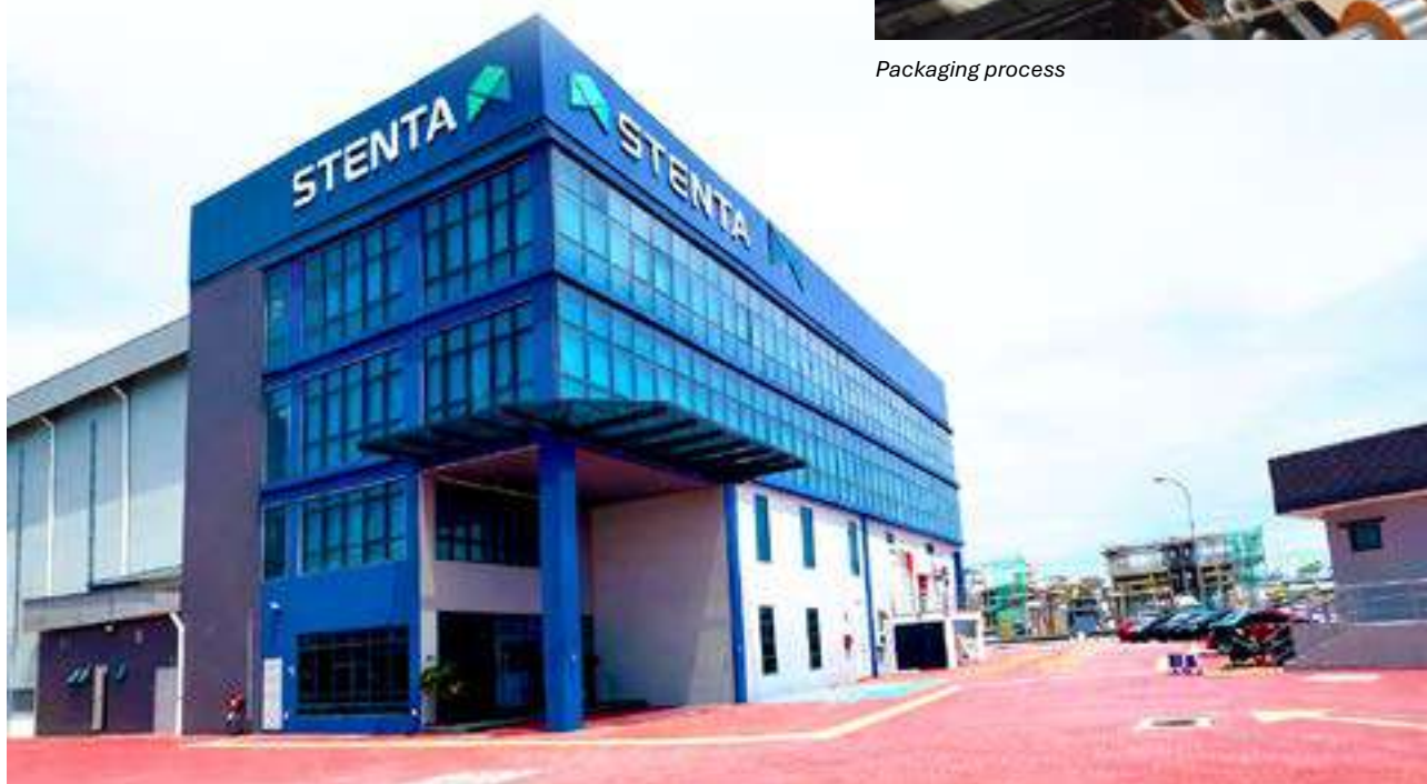
STENTA building Location: Bandar Baru Bangi, Selangor
