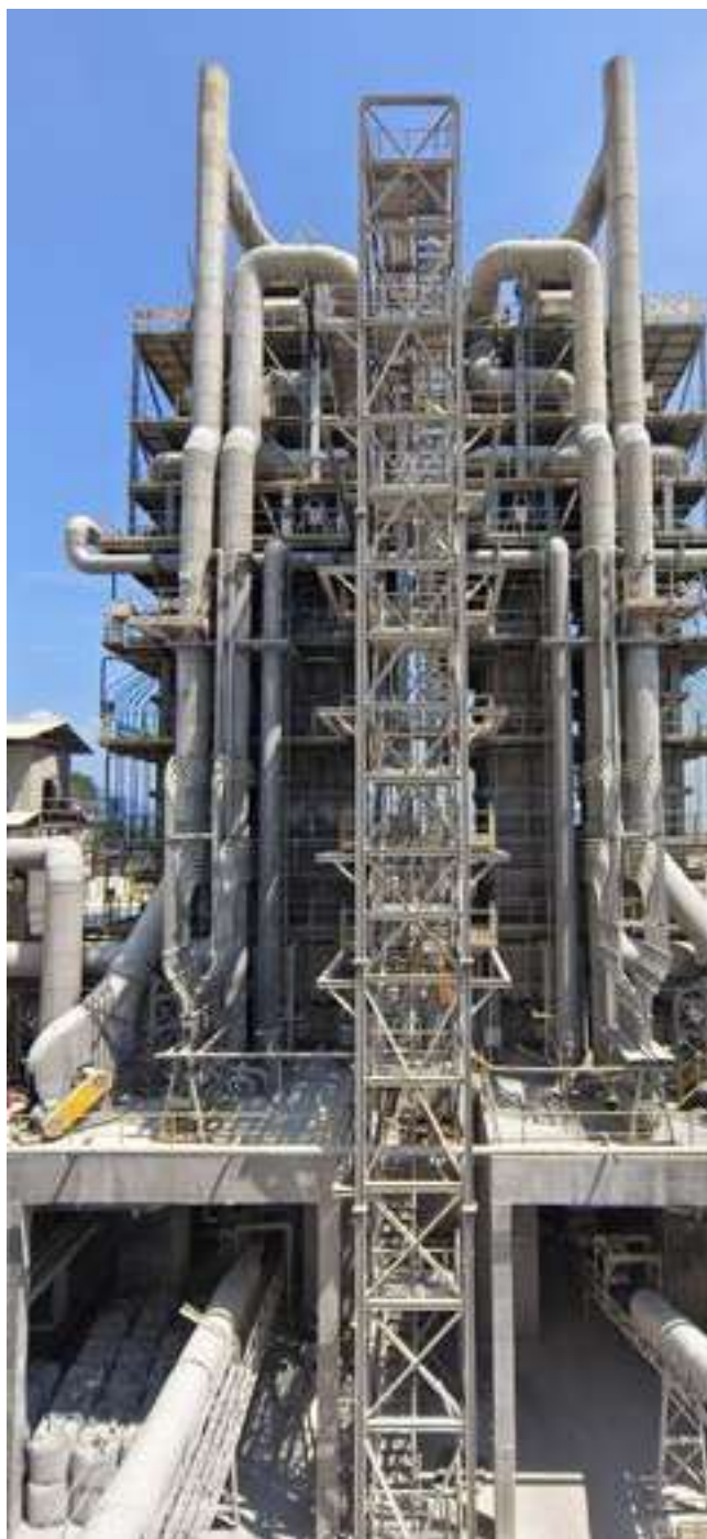
Lime Kiln Location: Gopeng, Perak
