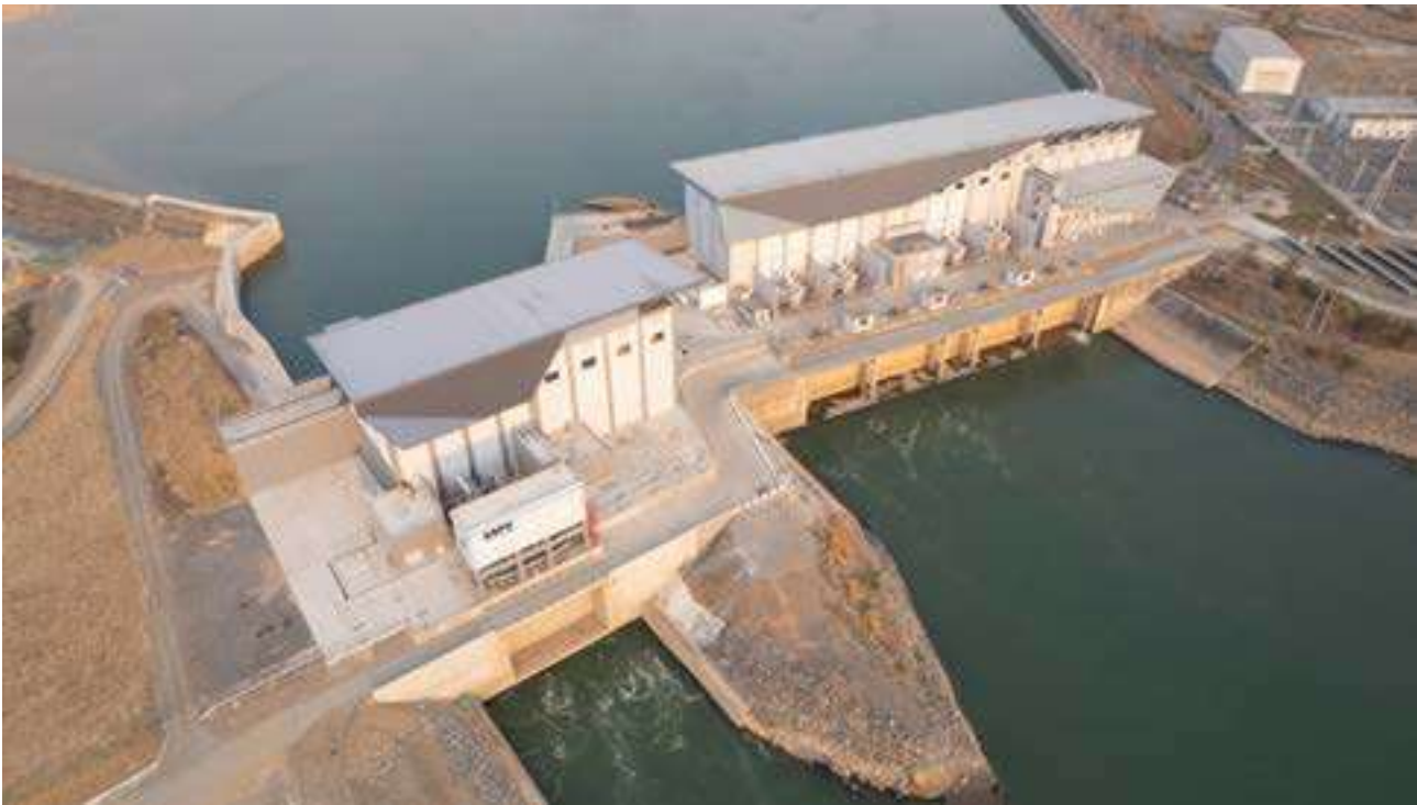
Hydropower Location: Don Sahong Hydropower Project, Laos
