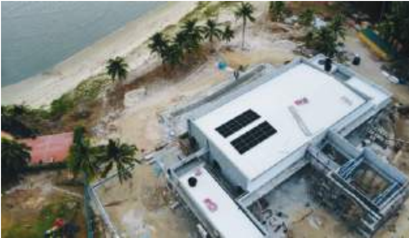
Solar system installed at SENJA in Ombak Villa Langkawi
