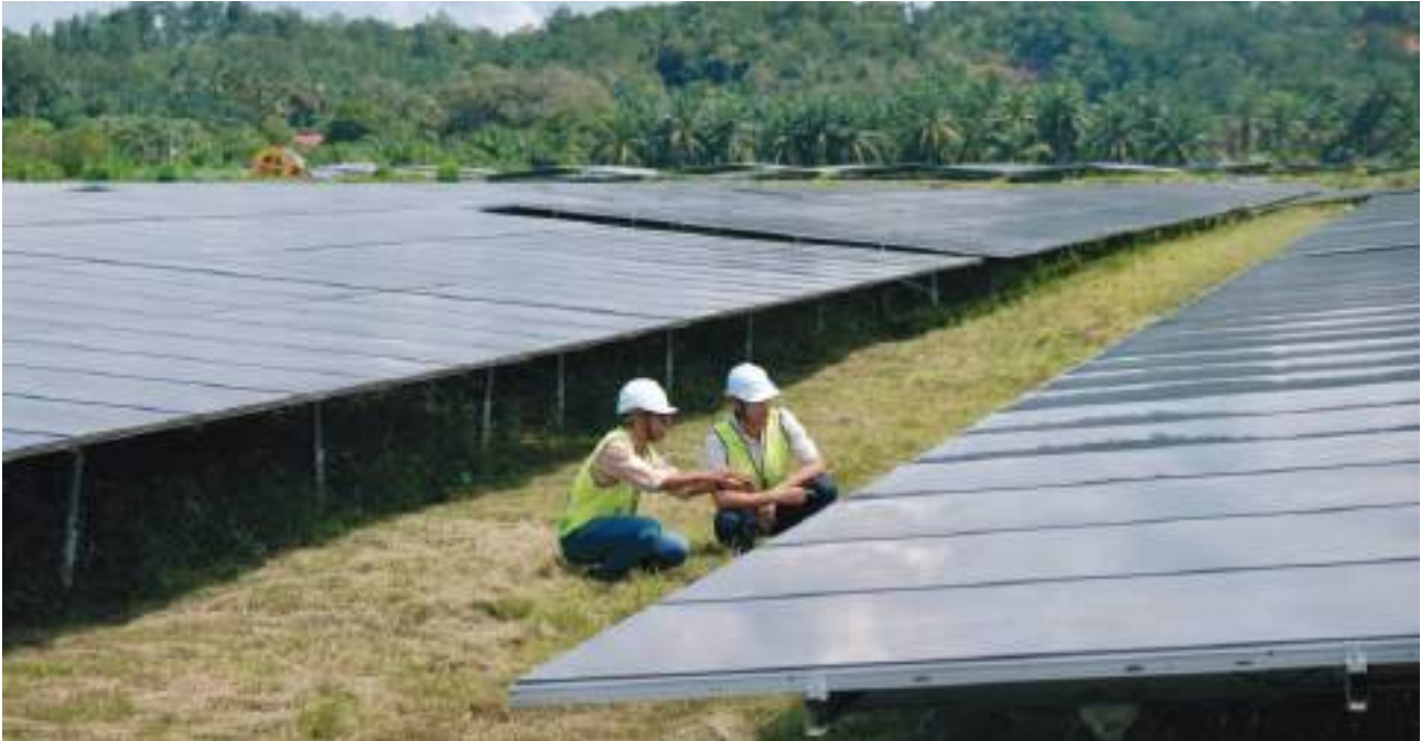
LSS4 Solar Photovoltaic Plant in Kerian, Perak
