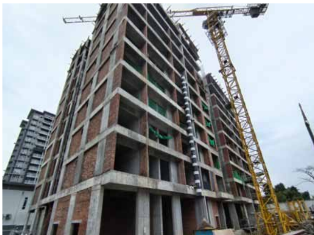
Proposed 128 Units of 17-Storey Condominium Skyvilla Block E, Kuching – Ongoing RC and Architectural works
