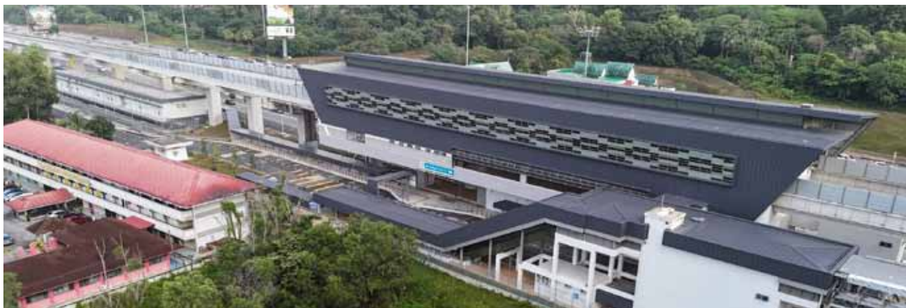
LRT3 GS01 Completion of Station, Viaduct and Parking Facilities at BU11 Station
