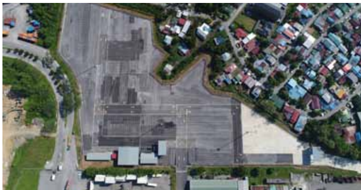
Completion of Phase 1 Vehicle Yard and Associated Facilities at Senari Port, Kuching
