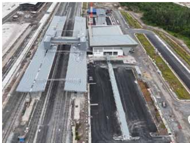
Ariel View of completed Station Works at ECRL Chukai Station, Terangganu
