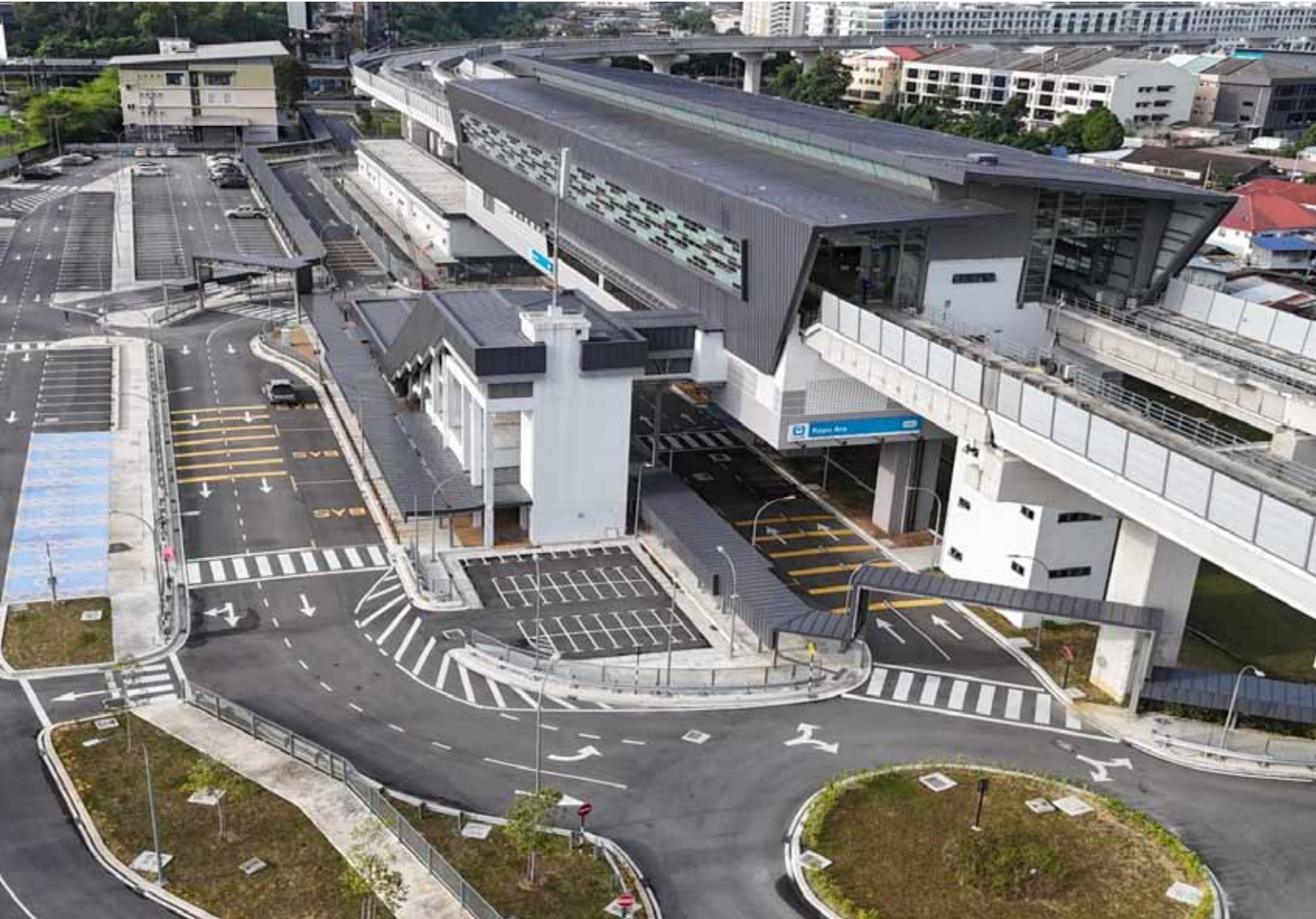
LRT3 GS01 Completion of Station, Viaduct and Parking Facilities at Kayu Ara Station.
