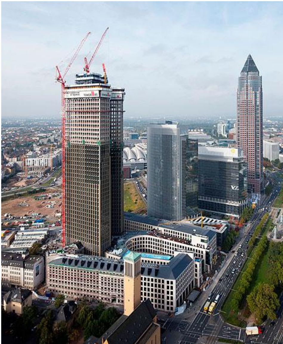
FRANKFURT, construction site of Tower 185
