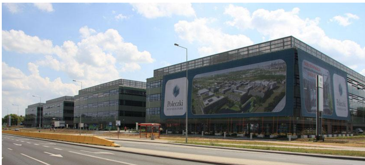
WARSAW, Poleczki Business Park, construction phase 1
