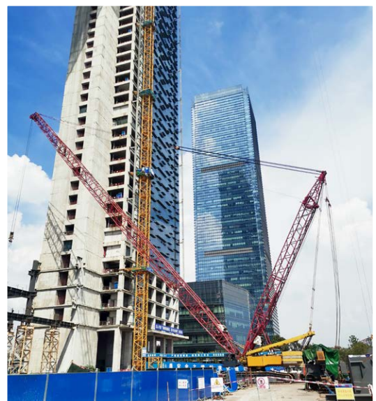
LOCATION: China EQUIPMENT: 250 Tonnes Crawler Crane SCOPE OF WORK: Equipment Rental
