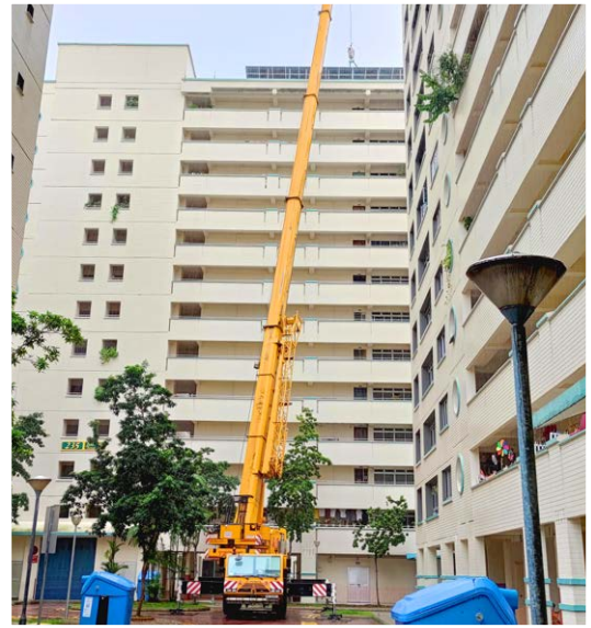
LOCATION: Singapore EQUIPMENT: 100 Tonnes Mobile Crane SCOPE OF WORK: Heavy Lifting Services
