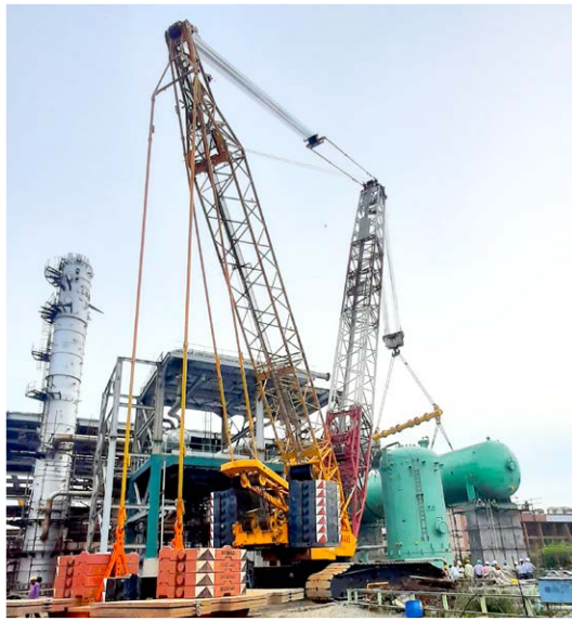
LOCATION: India EQUIPMENT: 600 Tonnes Crawler Crane SCOPE OF WORK: Heavy Lifting Services
