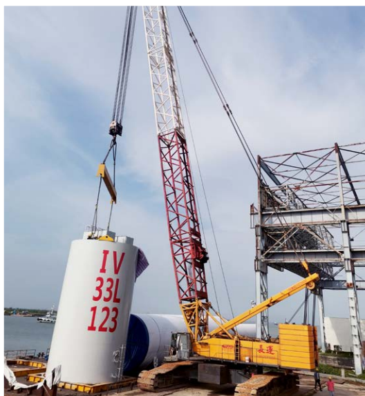
LOCATION: China EQUIPMENT: 550 Tonnes Crawler Crane SCOPE OF WORK: Equipment Rental
