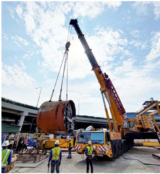
LOCATION: Singapore EQUIPMENT: 500 Tonnes Mobile Crane SCOPE OF WORK: Heavy Lifting Services
