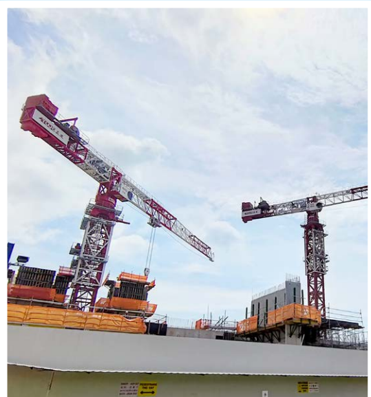
LOCATION: Singapore EQUIPMENT: 64 Tonnes Tower Cranes SCOPE OF WORK: Heavy Lifting Services
