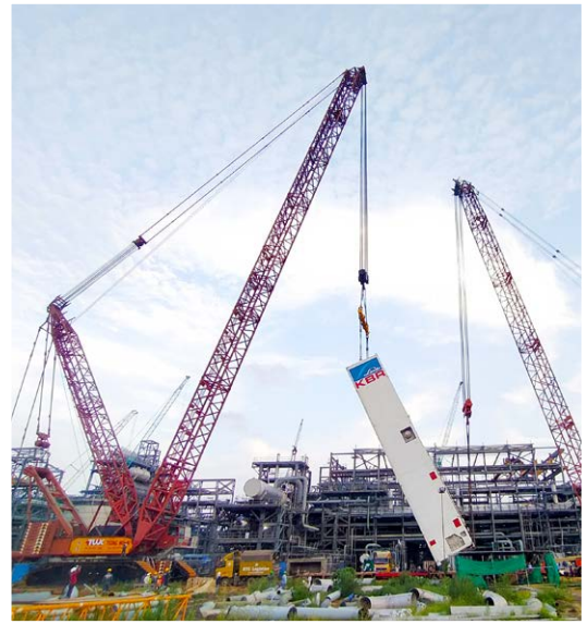
LOCATION: India EQUIPMENT: 1,250 Tonnes Crawler Crane SCOPE OF WORK: Heavy Lifting Services
