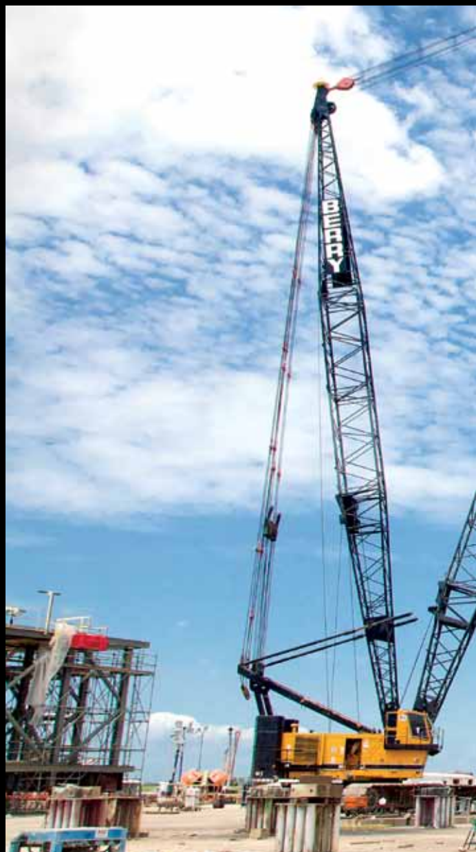
Above: Constructing the MOPU at the Gulf Cooper Shipyard, Galveston USA. The MOPU has been converted from an existing jack-up rig. With a processing module capable of producing 50,000 bopd.
