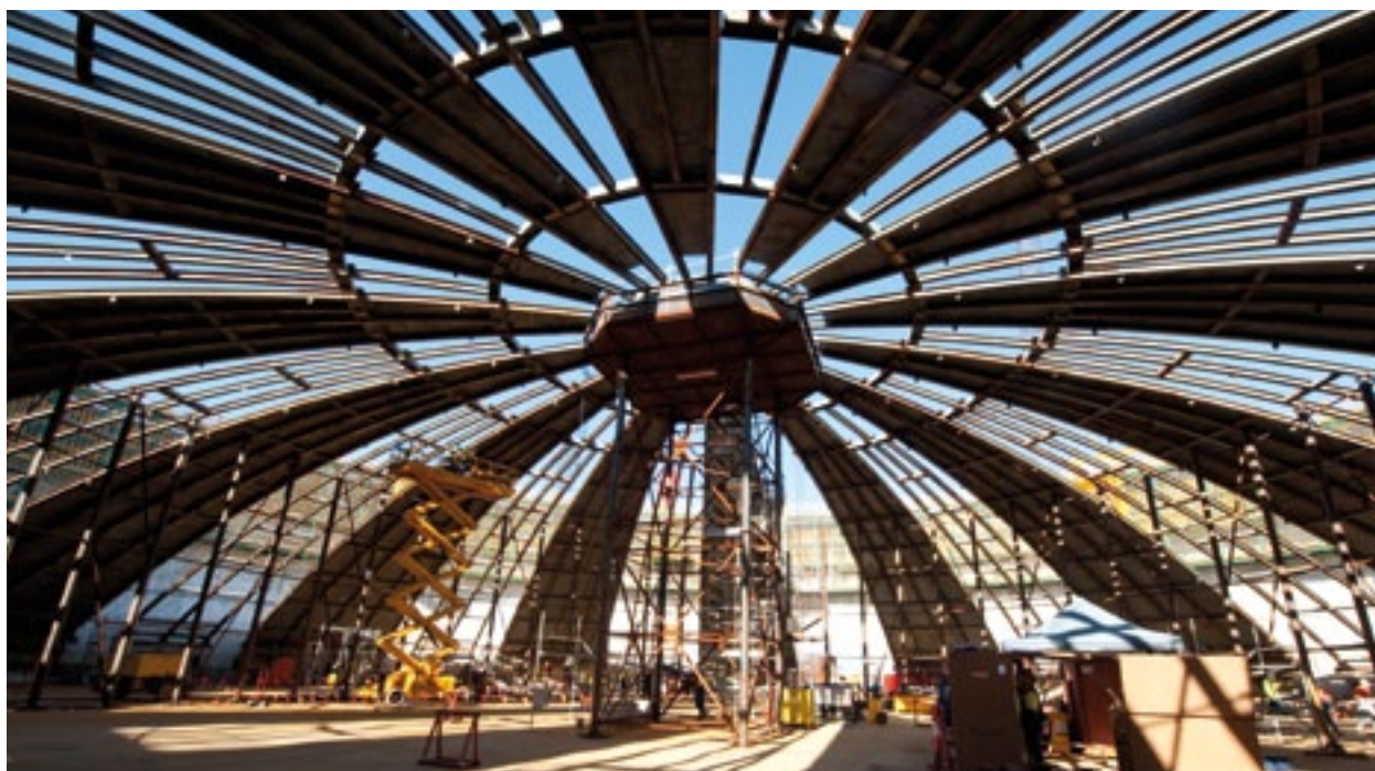
QCLNG terminal, Curtis Island, Australia Constructing one of the LNG storage tanks.
