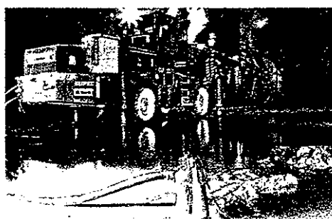
Inset above: 2 stage well point dewatering during the construction of an underpass on the main Dubai to Abu Dhabi road. Inset left: Strict legislation and safe working standards are met by Sykes electric submersible pumps in mines and tunnels. Below: Ten 16 inch high performance pumps overpumping the King Abdulla Canal, Jordan.
