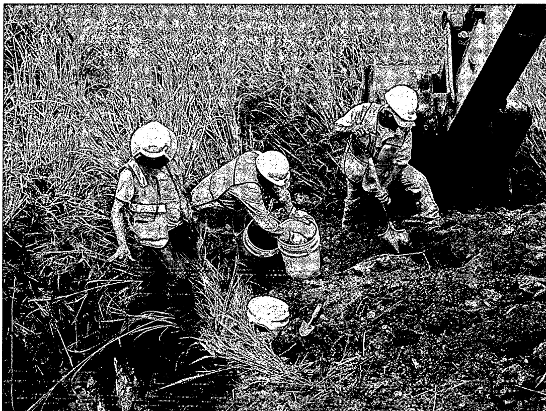
TSF ground Investigation test pit LIPT042 on the northern drainage channel above the main dam.
