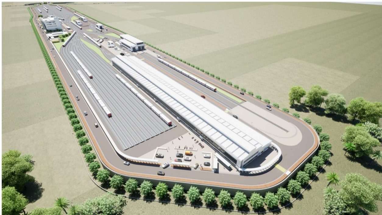
Perspective of the SCRIP-07 Projects- Earthworks and Underpass Works
