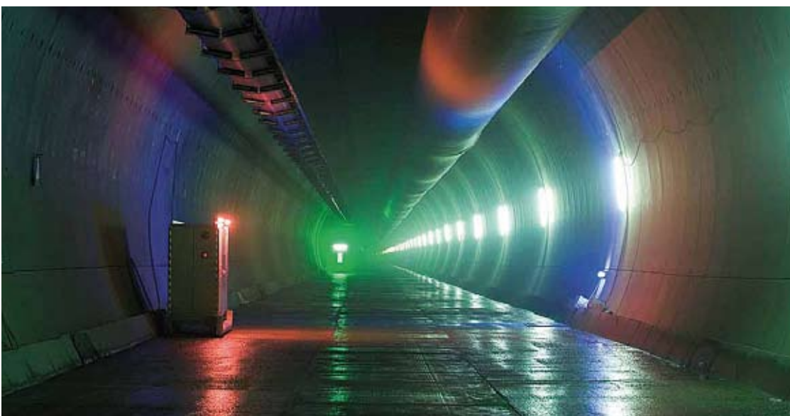
ISLISBERGTUNNEL, UETLIBERG WESTERN KNONAU, SWITZERLAND
