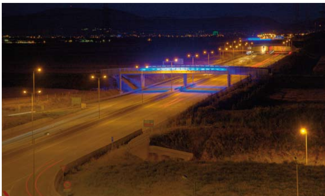
EXPRESSWAY S1, SCHWECHAT/RANNERSDORF, AUSTRIA
