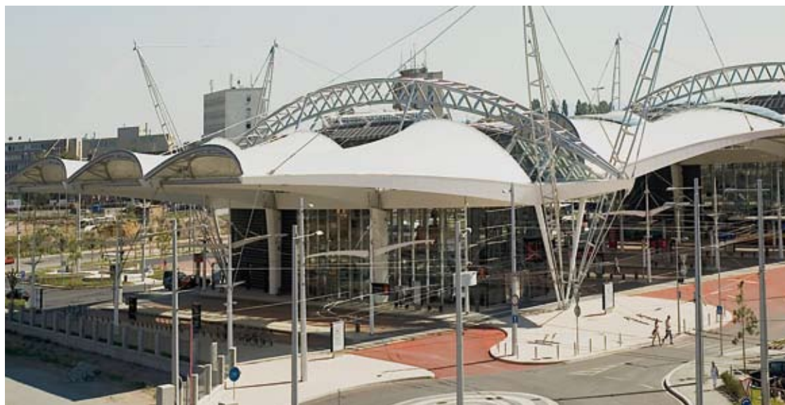
BUS TERMINAL HRADEC KRÁLOVÉ, KAPLICE, CZECH REPUBLIC
