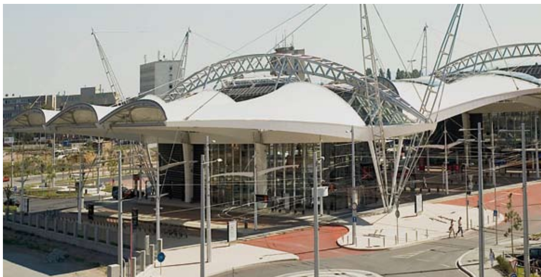
BUS TERMINAL HRADEC KRÁLOVÉ, KAPLICE, CZECH REPUBLIC
