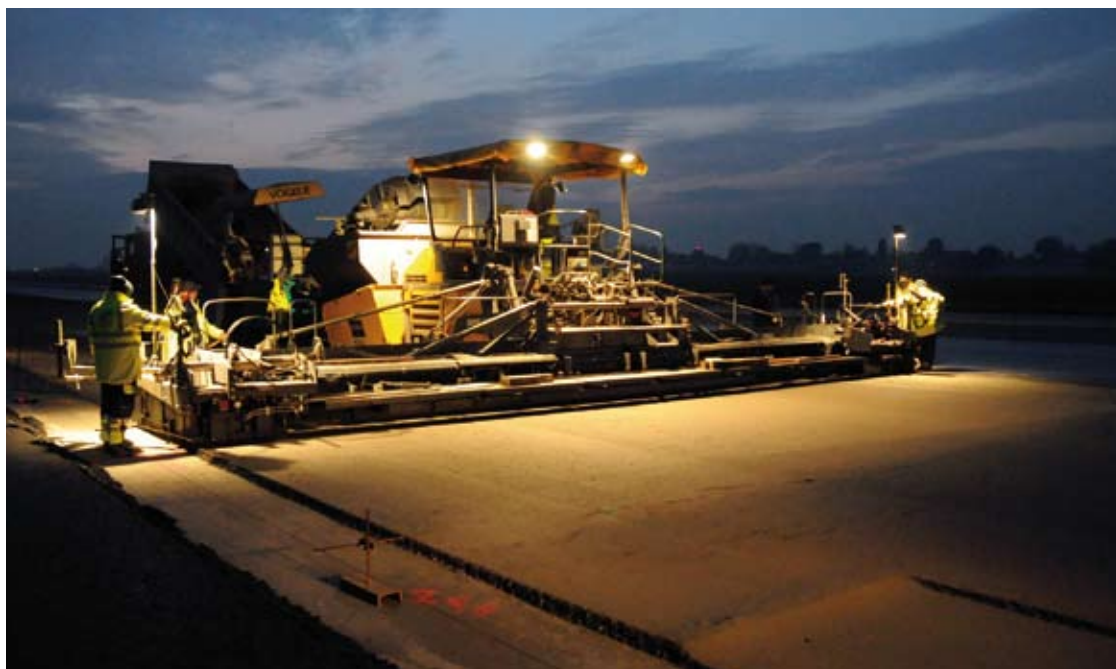
ASPHALTING AIRPORT KBALY, CZECH REPUBLIC
