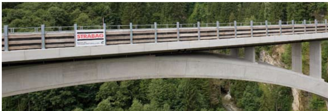
ANGER GORGE BRIDGE, BAD HOFGASTEIN, AUSTRIA
