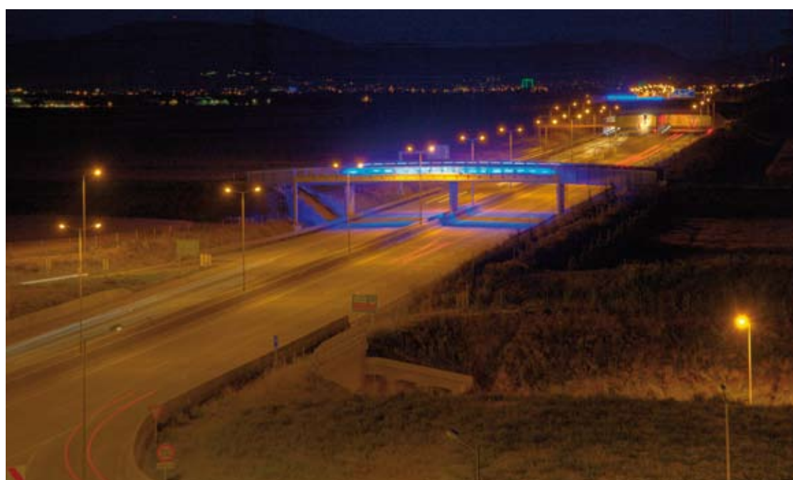
EXPRESSWAY S1, SCHWECHAT/RANNERSDORF, AUSTRIA
