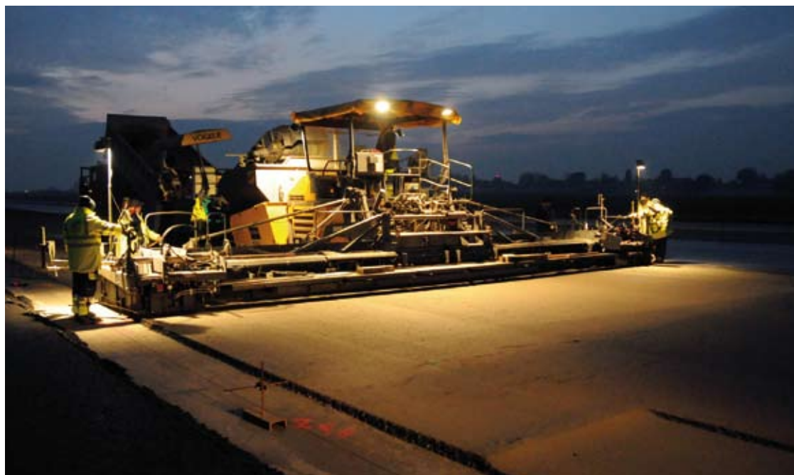
ASPHALTING AIRPORT KBALY, CZECH REPUBLIC
