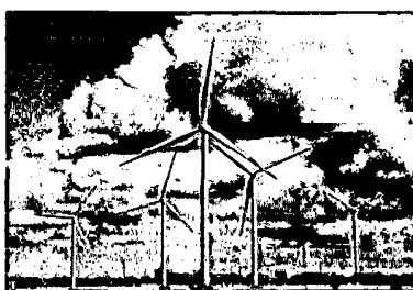
China Hebei Province Wind Farm
