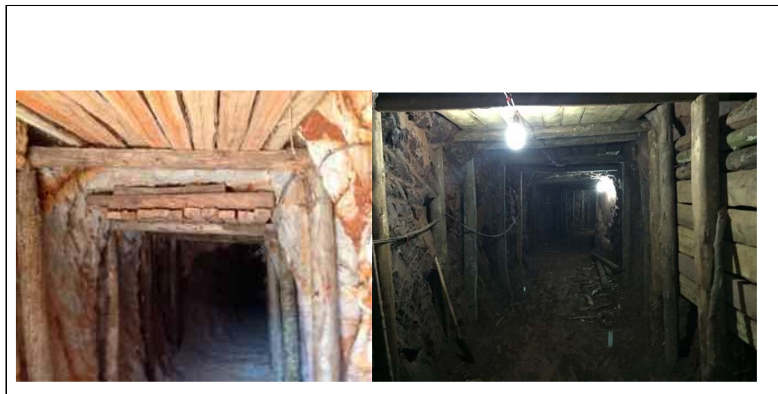
Figure 59: Examples of Tunnel Support
