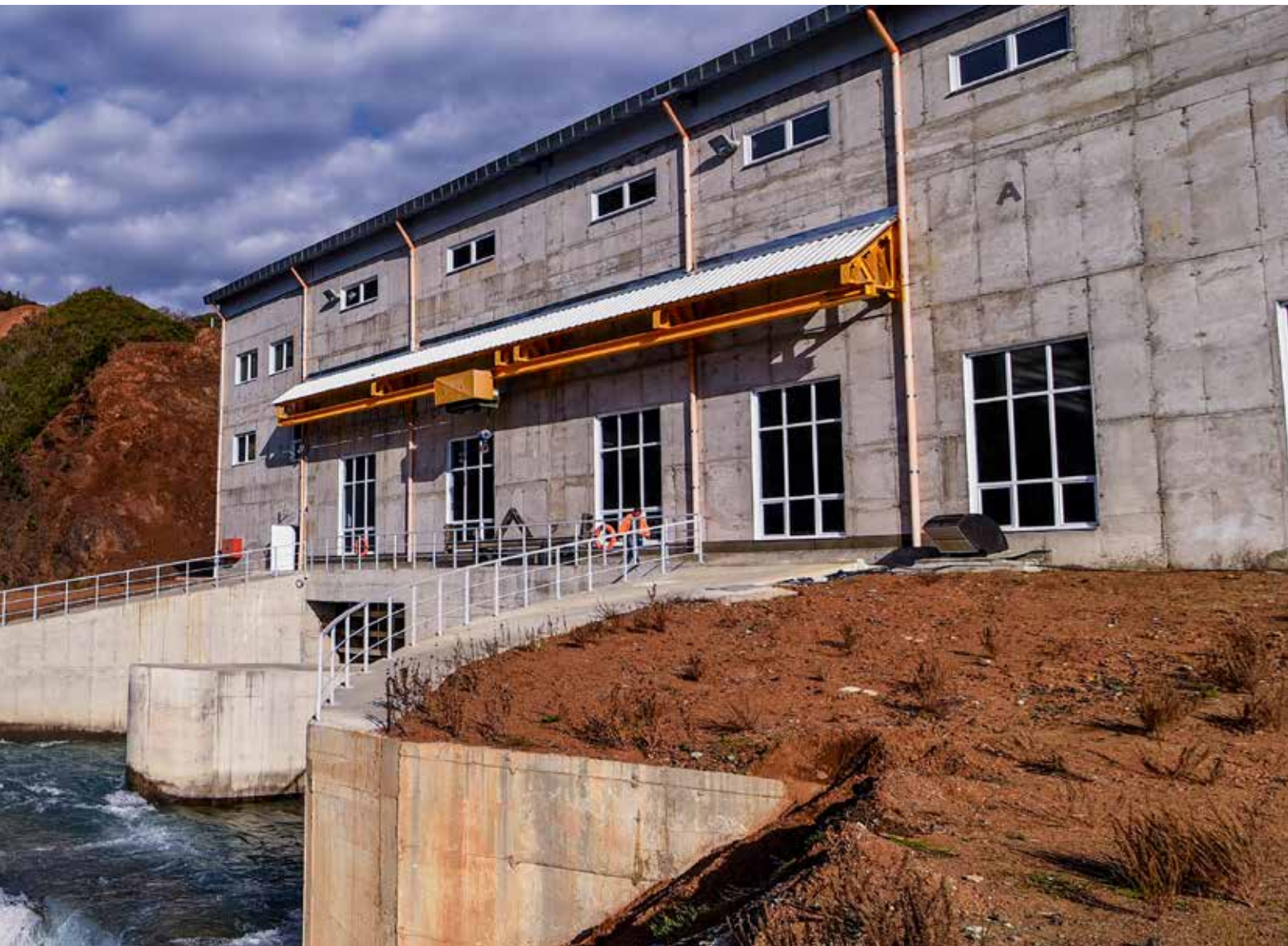
Peshqeshit HES / Peshqeshit HEPP
