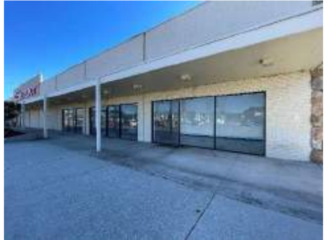
Front View of The Existing Building
