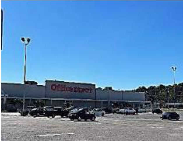
Front View of The Existing Building
