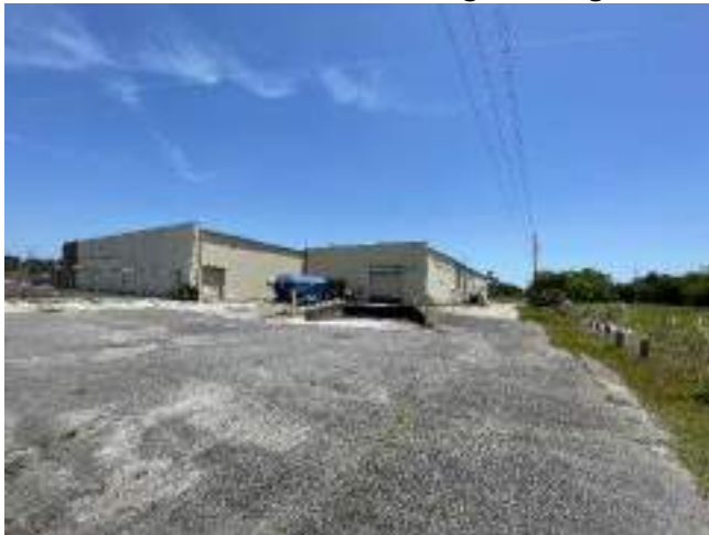
Back View of The Existing Building
