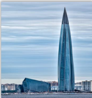
Gazprom Lakhta Center
