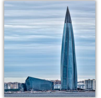
Gazprom Lakhta Center
