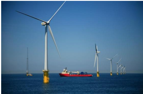
Fecamp Off-Shore Wind Farm
