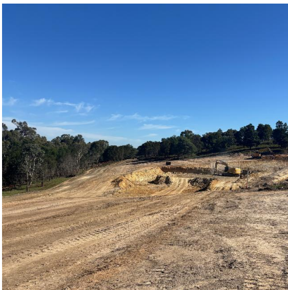
Figure 1. Box cut earthworks, 30 April 2026.
