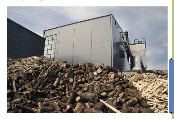
On the industrial estate of Kaiserbaracke, 4Energy Invest has developed a biomass cogeneration plant in cooperation with three local industrial parties, who produce finished or half-finished wood products for different industrial purposes. 4Energy Invest uses the wood waste it purchases from these partners as fuel and sells thermal energy to them. The produced electricity is fed into the distribution grid and sold to energy suppliers. The green benefits are sold to energy suppliers.
