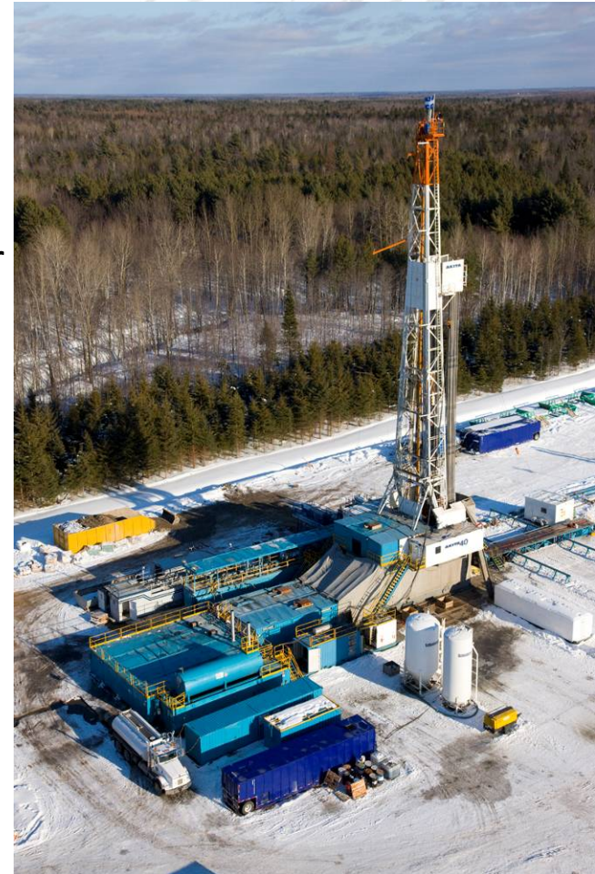
Drilling operations on Gentilly No. 2 horizontal
