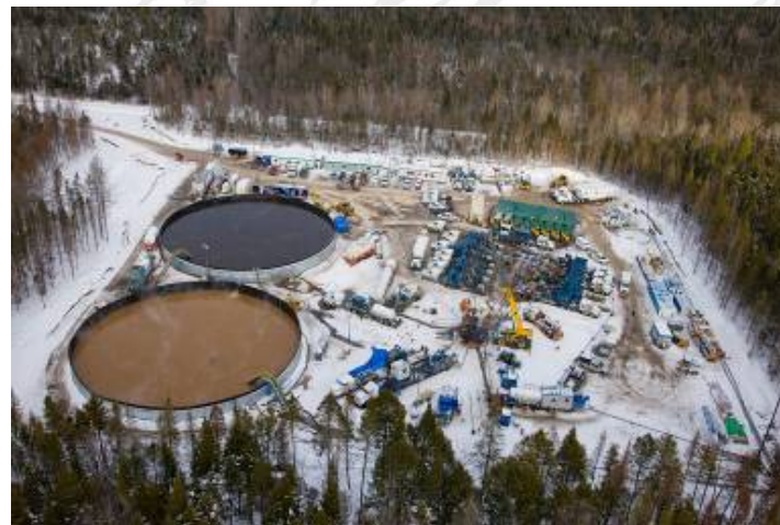
Frac completion operations on St. Edouard No. 1A horizontal
