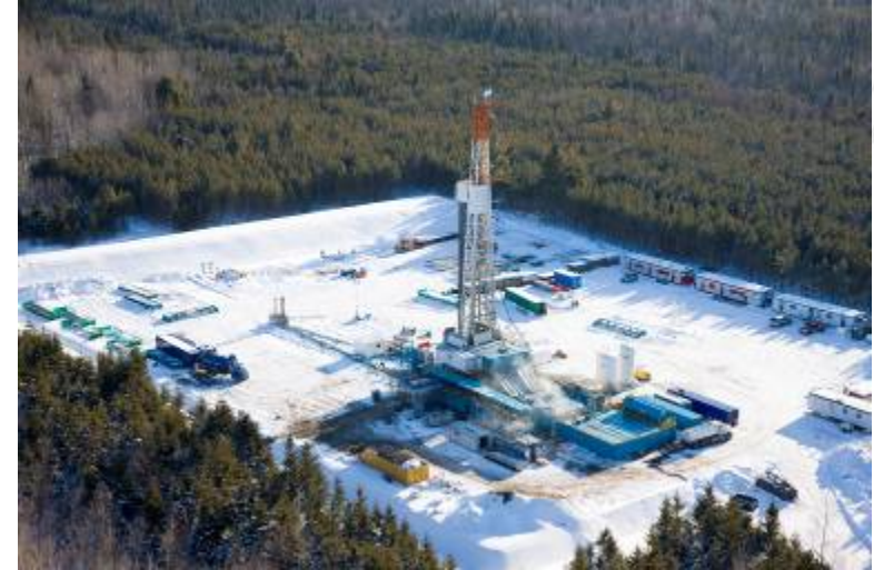
Drilling operations on Gentilly horizontal well
